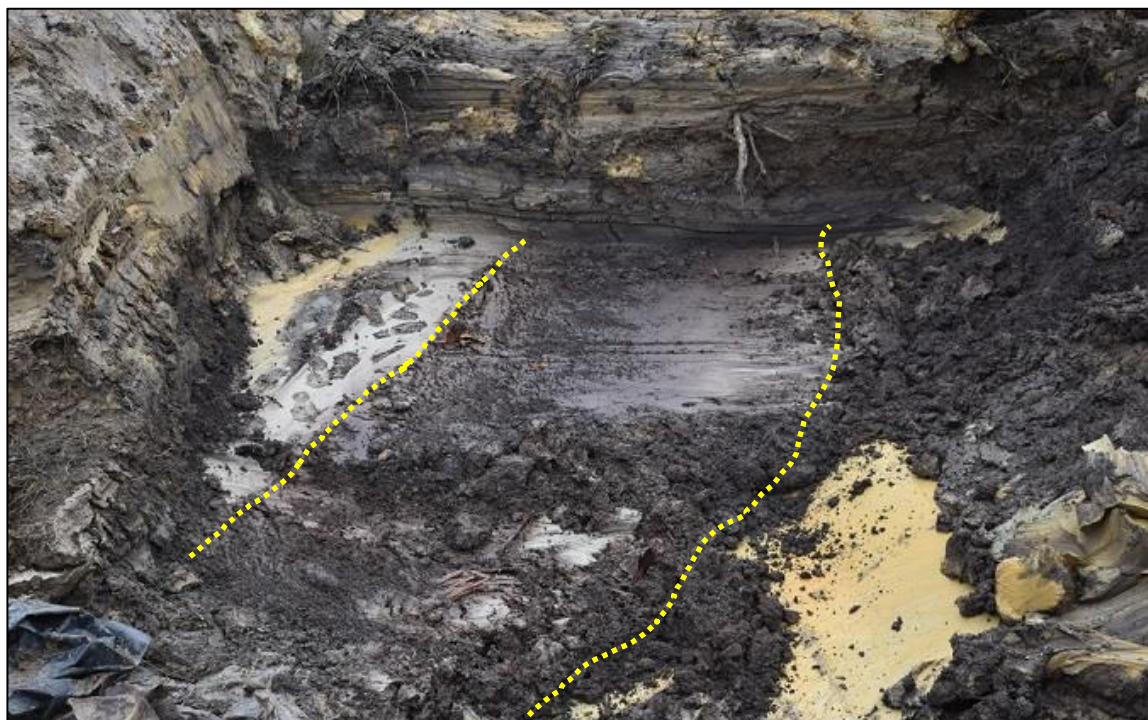
Figure 3.104 The extent of the palaeochannel (dashed lines) that was exposed within the drainage works at the Carran Road site
