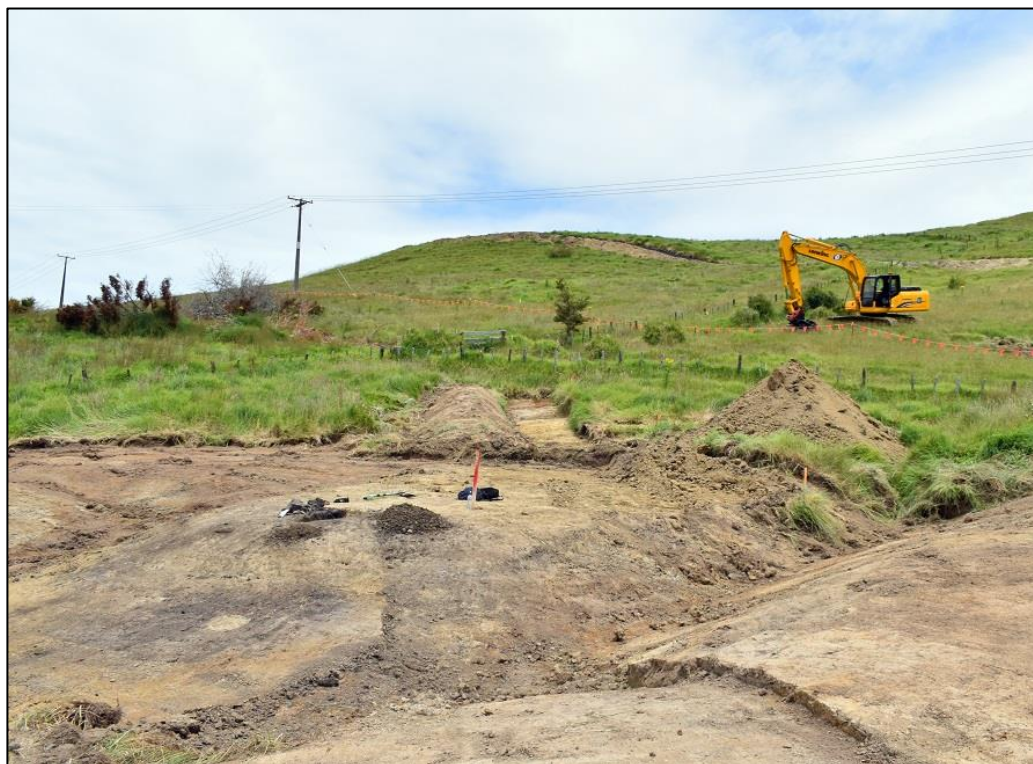
Figure 3.40 Southwest facing view showing the location of R10/1501 on a small terrace at the end of a historical landslip that would have descended downslope from the area behind the mechanical excavator. Scale: 0.5m
