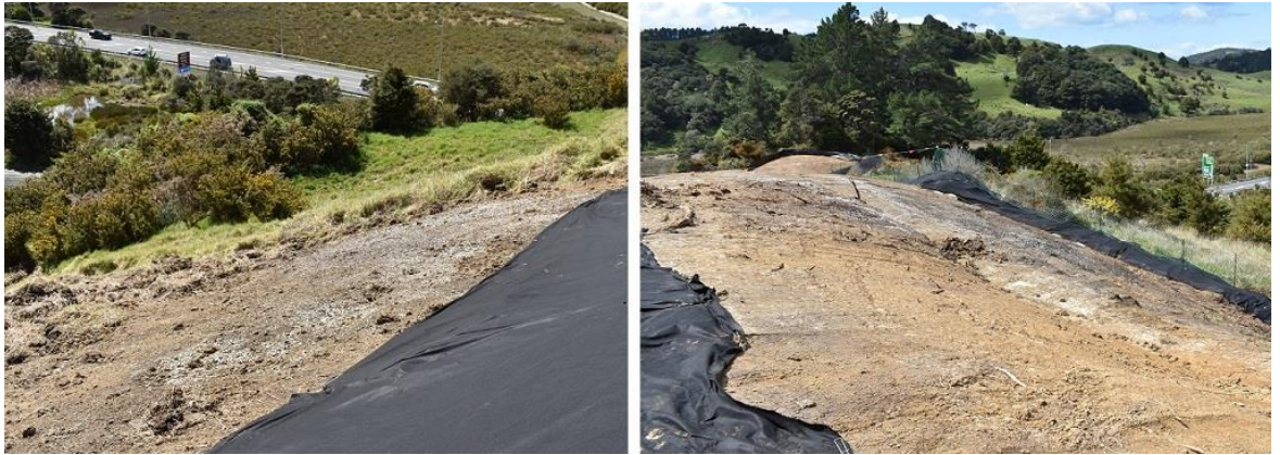
Figure 3.69 Slumping of the ridge spur to the north (left) and south (right) of the upper terrace of site R10/1106, with shell midden visible spilling down both slopes
