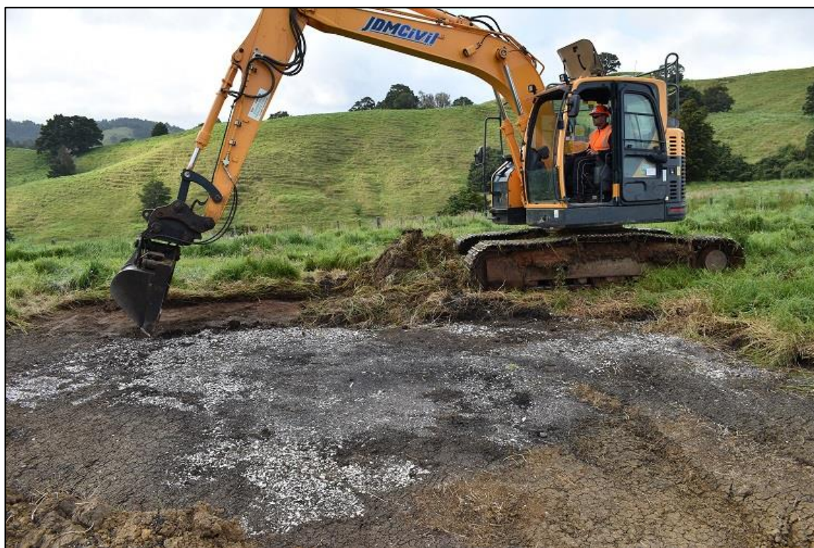
Figure 4.53 South-southwest facing view as the topsoil was stripped from the site exposing the midden deposit (1050)
