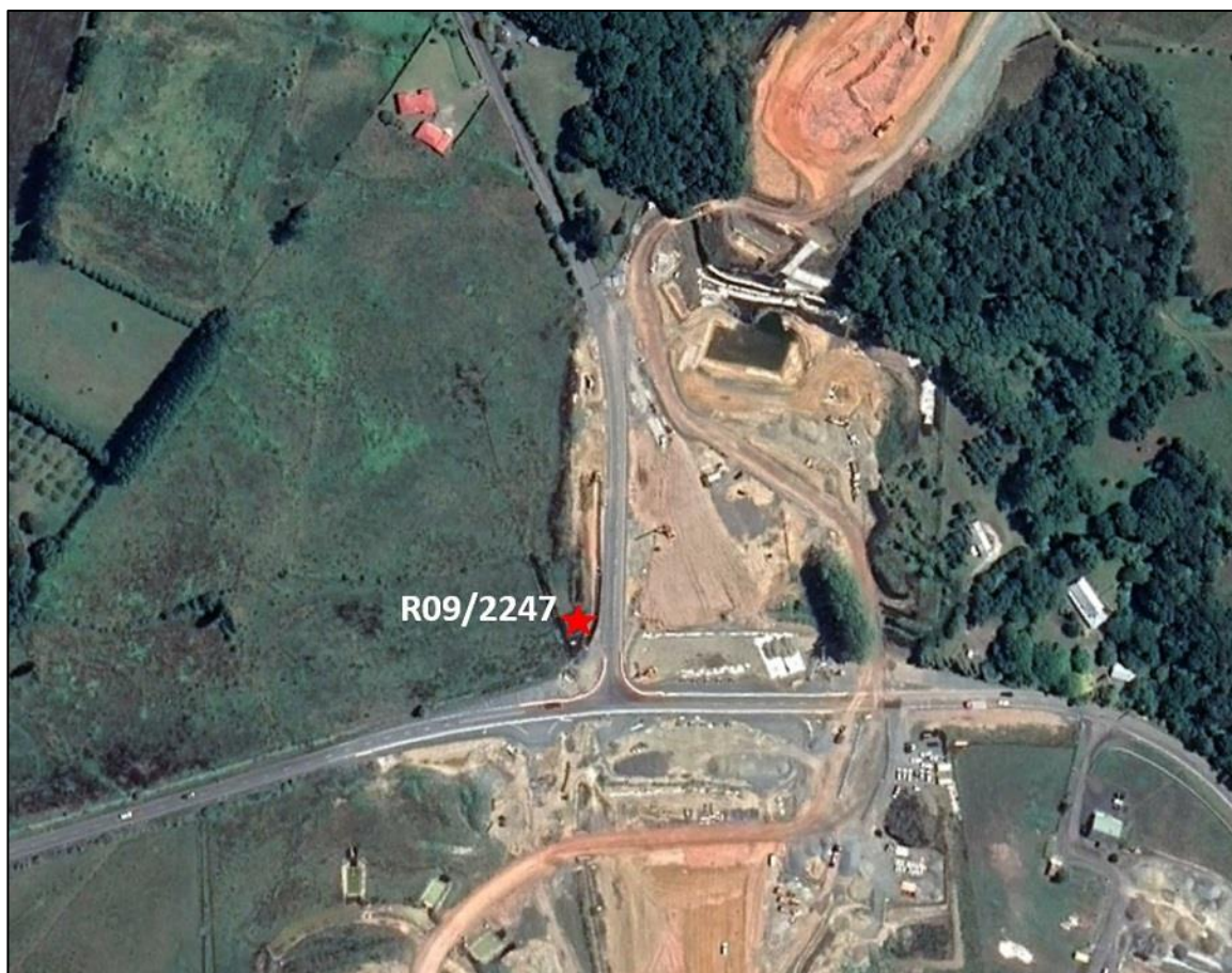
Figure 3.100 Location of site R09/2247 (wooden artefacts cache) close to the junction between Carran Road (running north from centre) and Woodcocks Road (bottom)
