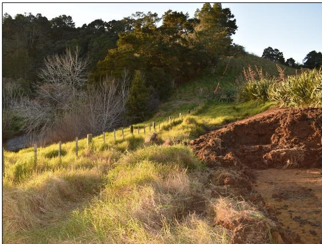
Figure 3.93 View facing north showing the silt bund excavation in which part of site R10/1510 was located. The Pūhoi River is just visible at centre left
